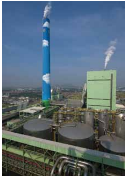
Overall view of alkali recovery system in Asia Symbol Shandong
