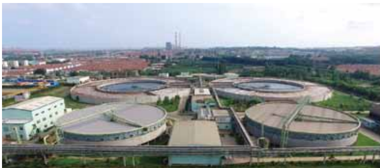
The cover constructed above the sewage treatment plant in Asia Symbol Shandong is to reduce the odor emissions
