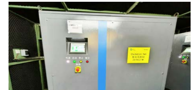
Energy-Saving Retrofit Project for Desulfurization and Oxidation Blowers
