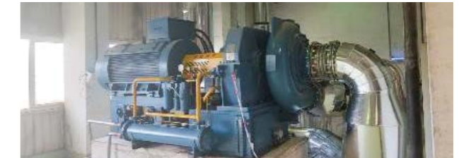
Vacuum System Retrofit Project
