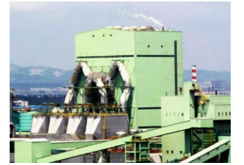
Alkali recovery boiler denitration system
