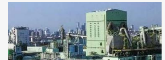
Upgrade and Renovation Project for Denitrification Process in Alkali Recovery Boiler
