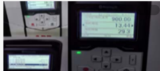
Variable Frequency Drive Retrofit for Cooling Tower Fans and Sludge Return Pumps
