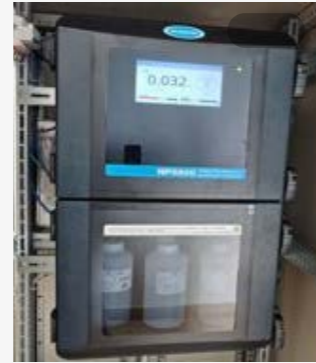
Online Monitoring Upgrade and Renovation of Effluent Discharge Outlets
